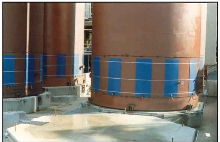
48 by 18 inch, type EGLX 500 Heating Panels, installed on 16 ft diameter, mild steel surfactant tanks to maintain a constant temperature of 130° F in minimum ambient temperatures down to -10° F. Photograph shows the heating panels banded directly to the tank surface in a vertical plane, prior to the application of 3 inch thick thermal insulation.
